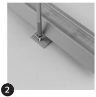
Position fixture and secure with screws (drill pilot holes where necessary).
